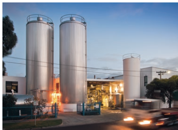
COBURG 10-16 Allenby Street Coburg VIC 3058 Australia
