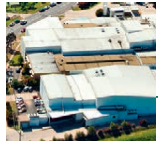
BEGA HEAD OFFICE AND PROCESSING & PACKAGING PLANT 23-45 Ridge Street North Bega NSW 2550 Australia
