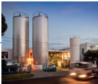
COBURG 10-16 Allenby Street Coburg VIC 3058 Australia
