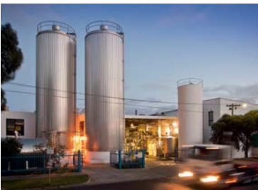
COBURG 10-16 Allenby Street Coburg VIC 3058 Australia
