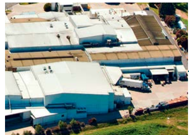
BEGA HEAD OFFICE AND PROCESSING & PACKAGING PLANT 23-45 Ridge Street North Bega NSW 2550 Australia
